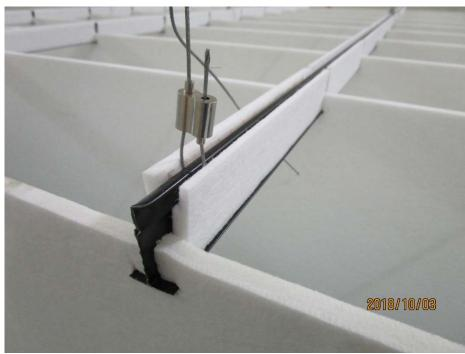
Figure 2 - Detail of baffle material, spacers, mounting method
